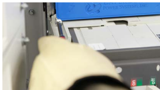
Screws Help Secure The Breaker
