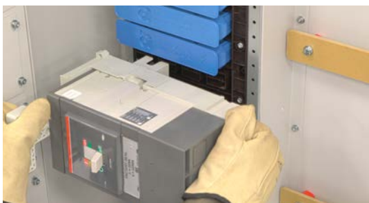
The Breaker Is Inserted Into The SafePanel
